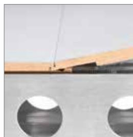
Simply place tongue and groove together at a slight angle, click into each other and press onto the aluminium frame.
